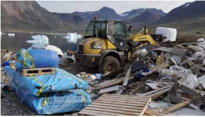
Dumping asbestos waste, photo Finn Larsen
